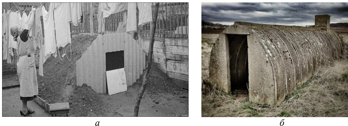
Fig.1. Shelters in Great Britain during the Second World War: a) Anderson's shelter; b) Stanton shelter made of precast concrete
