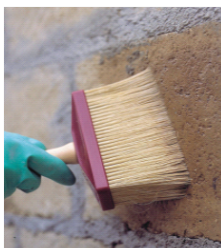
Pic 1. Consolidation of the base
