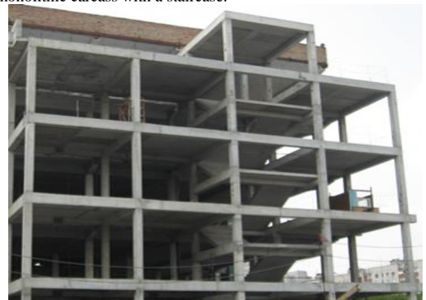
Fig.4: Reinforced concrete monolithic frame of the reconstructed building.
