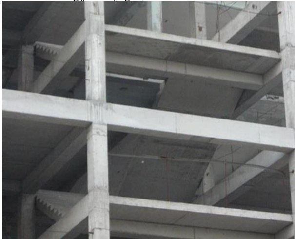
Fig. 5: A fragment of a reinforced concrete frame of a reconstructed building
