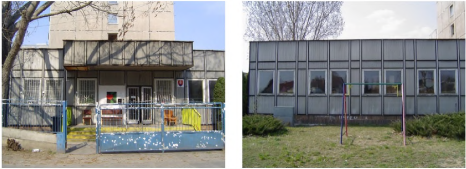
Fig.2. Center-shelter Bethany in Malacky town
