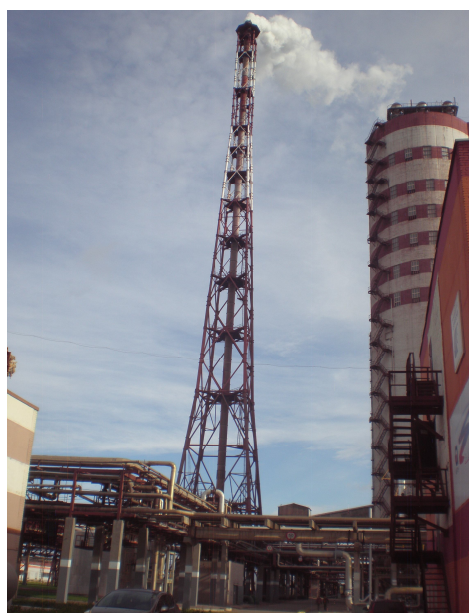
Fig. 1.- Metal exhaust pipe and bearing tower of the shop "Ammonia 4"
