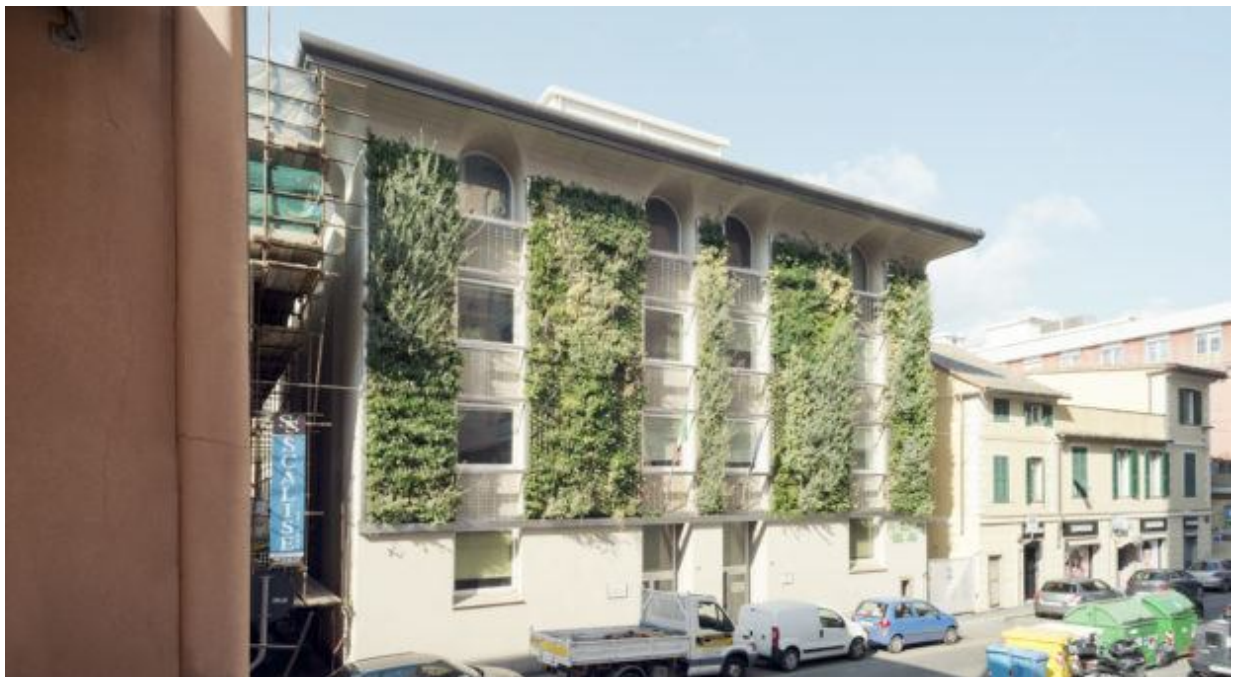
Fig. 4. Green Facade on a public institution office building, Genoa, Sestri Ponente, Italy
