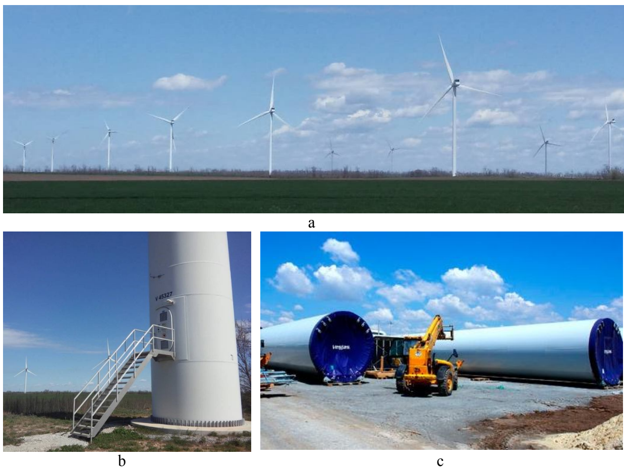
Fig. 3. Botievskaya Wind Power Station: a - wind generators; b - the lower part of the tower; c - montage of towers
